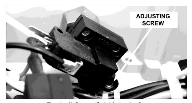
Fig. 10 – Air Pressure Switch in Junction Box
