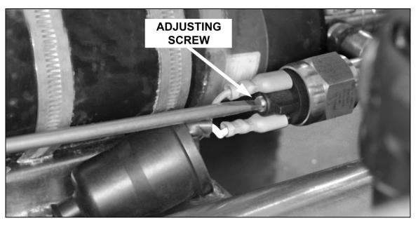
Fig. 11 – Pump Pressure Switch with Screwdriver
